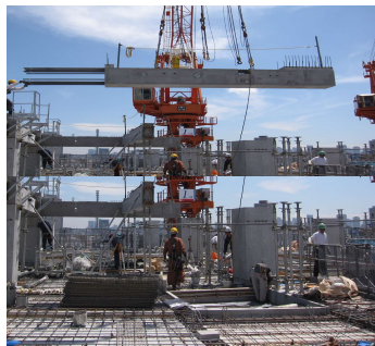
Rapid construction of high-rise building with precast technology
